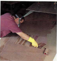
Don't spare the glue. A liberal amount of urea resin glue applied with a squeegee and roller guarantees a rigid bond at the glue-line.
